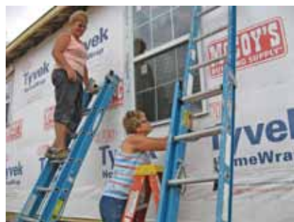
Marion and Helen installing a window.
